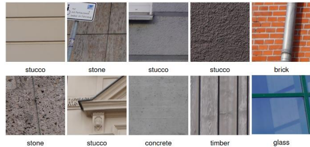
Fig. 4: Samples of 10 representative patches (out of 541 extracted), each with a size of 256 x 256 pixels, annotated with their identified material labels
