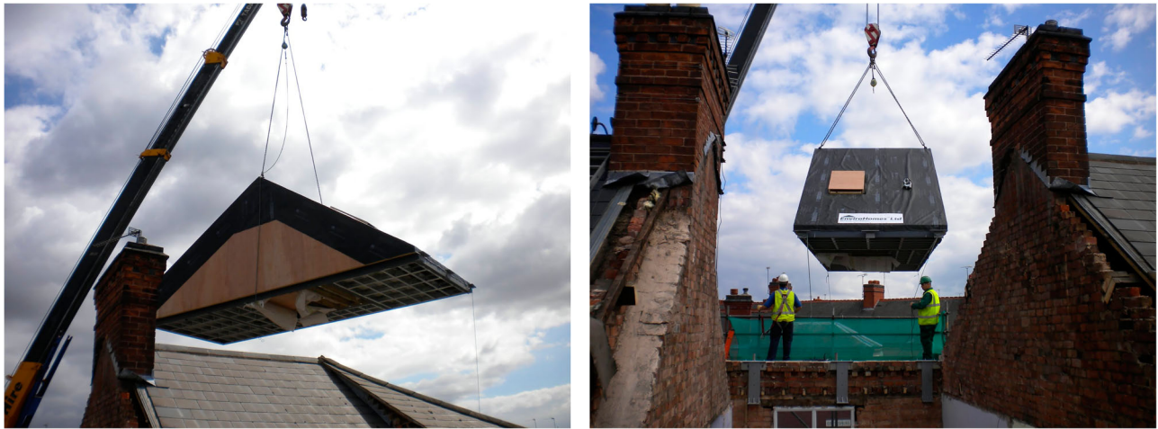
Figure 3. Roof pod installation on-site ('Retrofit for the Future', 2010).
