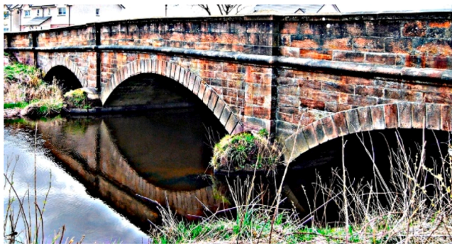
Fig. 2. Nith bridge, New Cumnock (Scotland).
