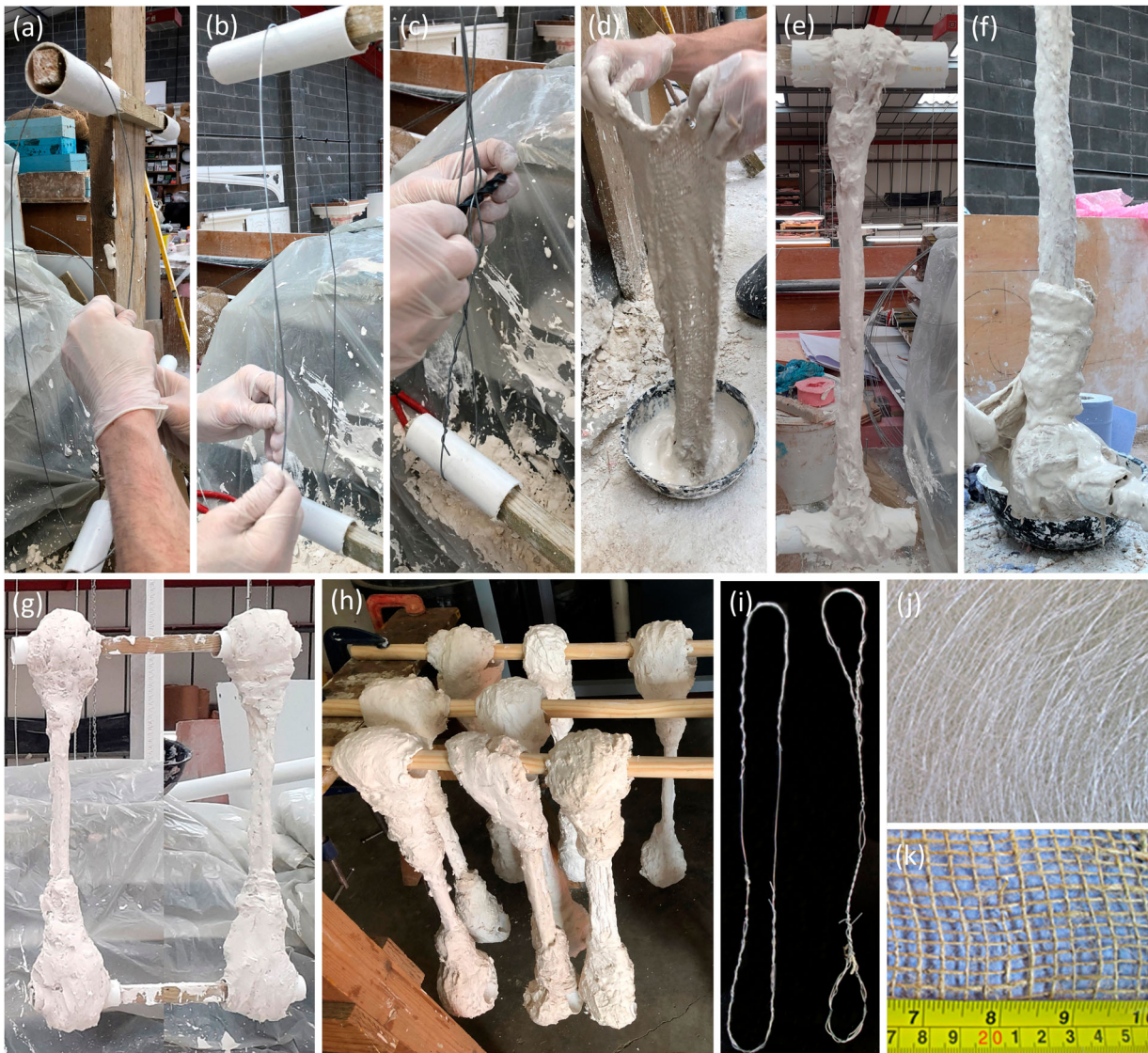
Figure 4. Typical steps in fibrous plaster wads fabrication within an industrial workshop environment: (a) Looping a 1.2 mm diameter steel wire length around two pipe lengths positioned on a bespoke timber frame; (b) Hand twisting the steel wire ends to form a loop of wire ('looped'); (c) Using a drill bit length as a tommy bar to twist the looped wire ('looped-twisted'); (d) Soaking hessian scrim with gypsum plaster; (e) Soaked scrim being wrapped and twisted around the steel wire to form a wad; (f) Extra soaked hessian wrapped around to strengthen ends around the eyelets and ensure wad failure occurs in the central section; (g) Completed test specimens curing; (h) Once cured, test specimens were stored prior to testing; (i) Wire specimens looped (left) and looped-twisted (right); (j) Continuous fibre glass (CFG) mat; and (k) Hessian scrim (jute fibres).
