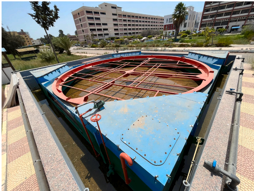
Fig. 4. The partially submerged photovoltaic prototype platform in the water basin deployed at the campus of Port Said University, Egypt.
