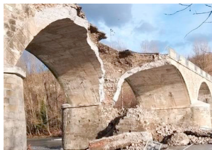
Fig. 3. Samone Bridge on Panaro River, Italy (photo courtesy of lapressa.it ).
