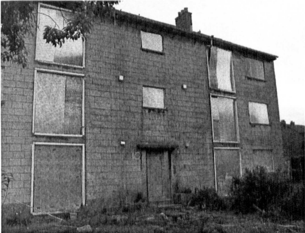
Figure 8: Original Easterhouse housing, prior to demolition.
