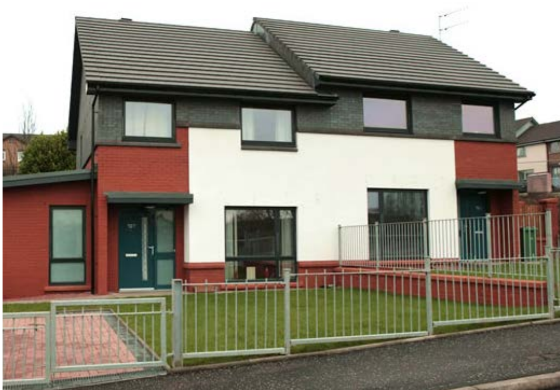
Figure 6: An example of Cernach Housing Association properties in Drumchapel, 2017.
