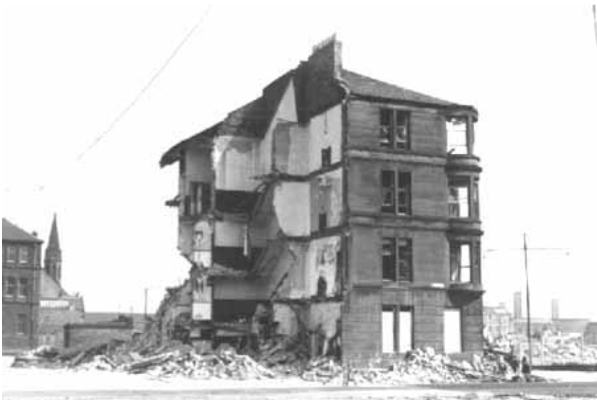
Figure 11: Demolition at Bernard Street, Bridgeton in the 1970s 32 .
