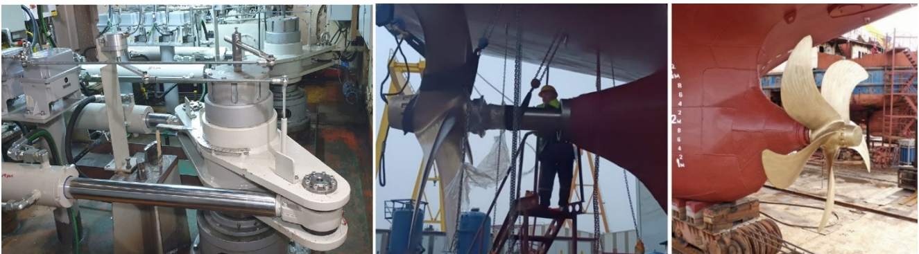
Figure 11. Installation of the new twin S/G system and shaft and propeller.
