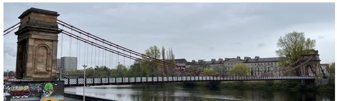
Fig. 2. South Portland Street Suspension Bridge (lat.: 55.854937, lon.: -4.255578).
