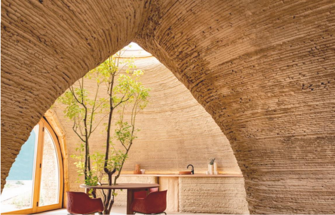
Figure 12. TECLA in Massa Lombarda, Italy. Credits: Iago Corazza Available at TECLA Technology and Clay 3D Printed House / Mario Cucinella Architects | ArchDaily
