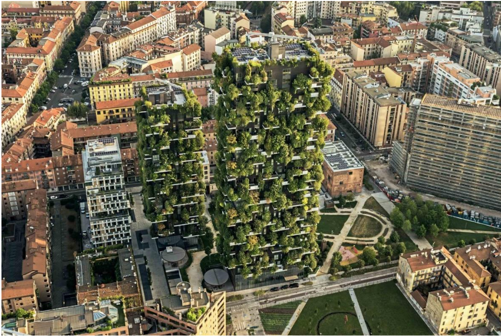
Figure 04, Bosco Verticale in Milan available from Vertical Forest | Milan | Stefano Boeri Architetti
