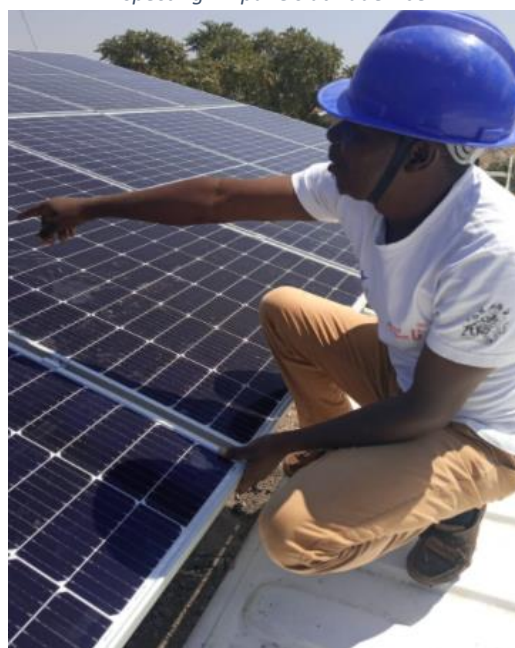
Inspecting PV panels at Kudembe
