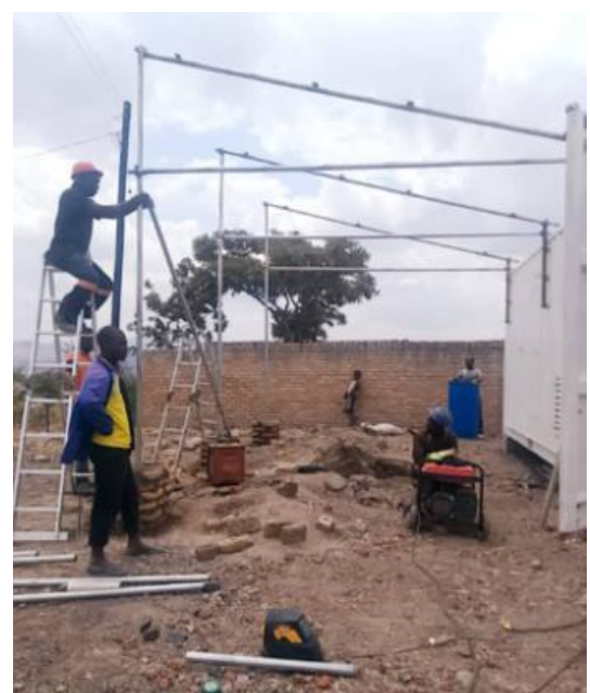
Construction of Kudembe generation hub
