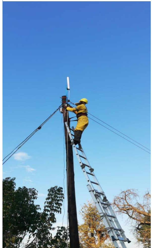
Maintenance activities on the distribution grid
