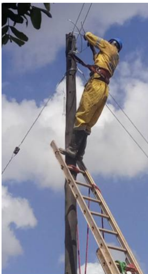
Distribution grid maintenance
