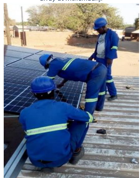
BNG Installation team commissioning PV array at Mthembanji
