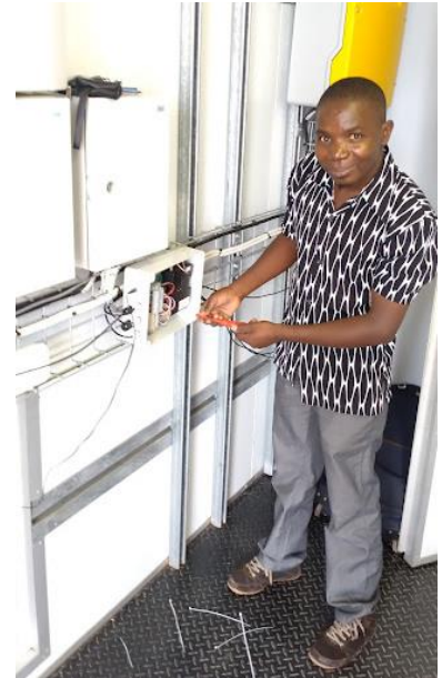
Installing the battery temperature monitor at Mthembanji
