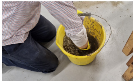
Step 2: Mixing the concrete to the right consistency
