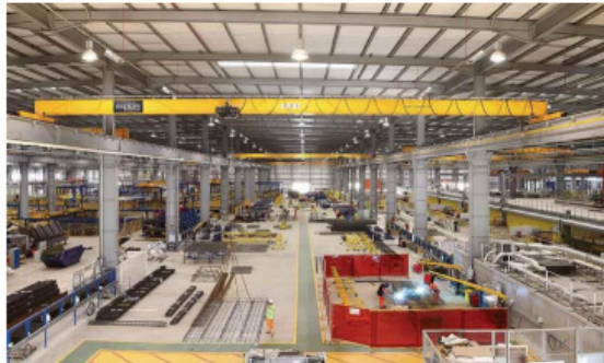
Construction Scotland Innovation Centre (overhead crane)
