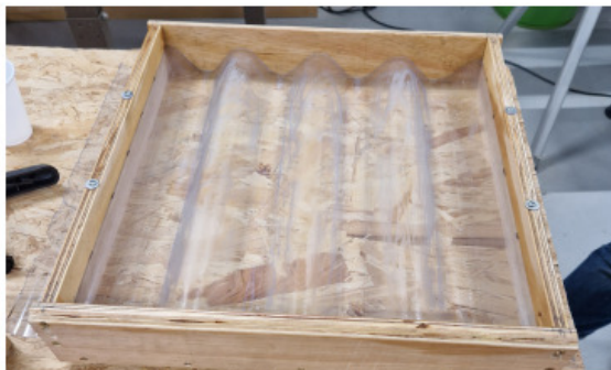
Step 1: Creating the shutter-work with corrugated plastic panel
