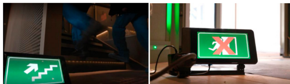
Figure 7. Dynamic exit signs.
