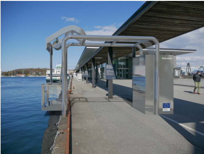
Figure 13: Draft layout of charging point for the Stavanger Demonstrator at Fiskepiren, Stavanger
