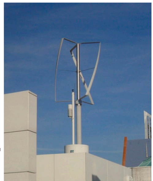
Fig. 6. Working principles and wind turbines installed at the rooftop of the building (a) Savonius [33,34] and (b) Darrieus [35,36].
