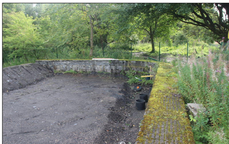
Figure 2. Treatment basin at Bowling prior to installation of geofabric.
