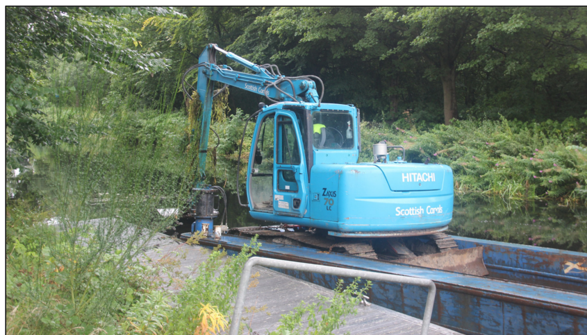
Figure 4. Barge-mounted excavator in operation on the Forth & Clyde Canal at Old Kilpatrick, September 2020.
