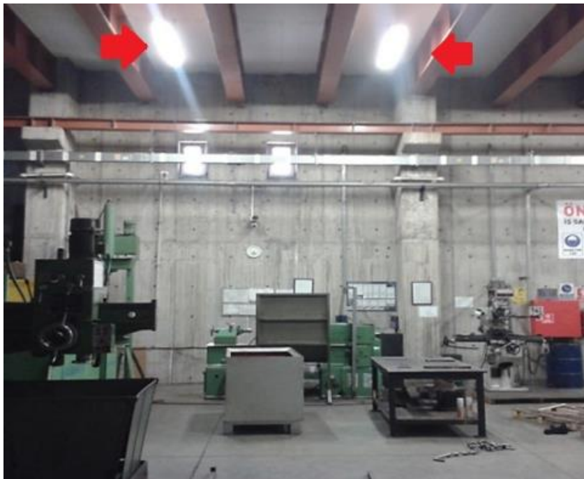
Figure 10: Unnecessary use of lighting in the machine shop of the case plant
