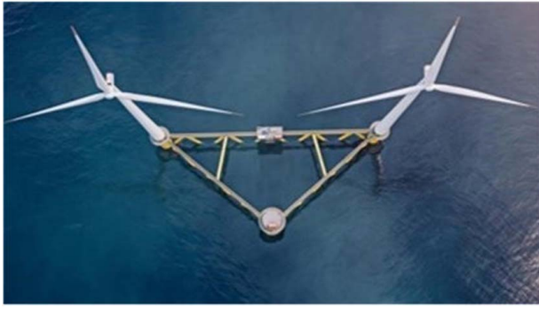
Fig. 1 Hexicon AB twin turbine concept
