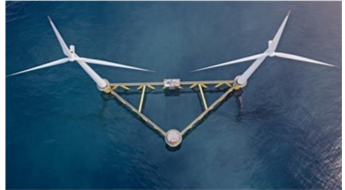
FIGURE 2. HEXICON AB TWIN TURBINE CONCEPT.
