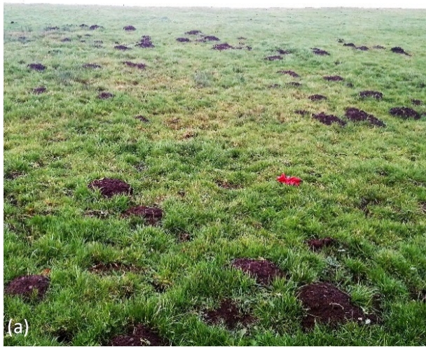
Figure 14: (a) Soil deposits on the west side of the downstream face of the dam. Slope instability on an areas located at (b) the toe of the dam and (c) towards the spillway.
