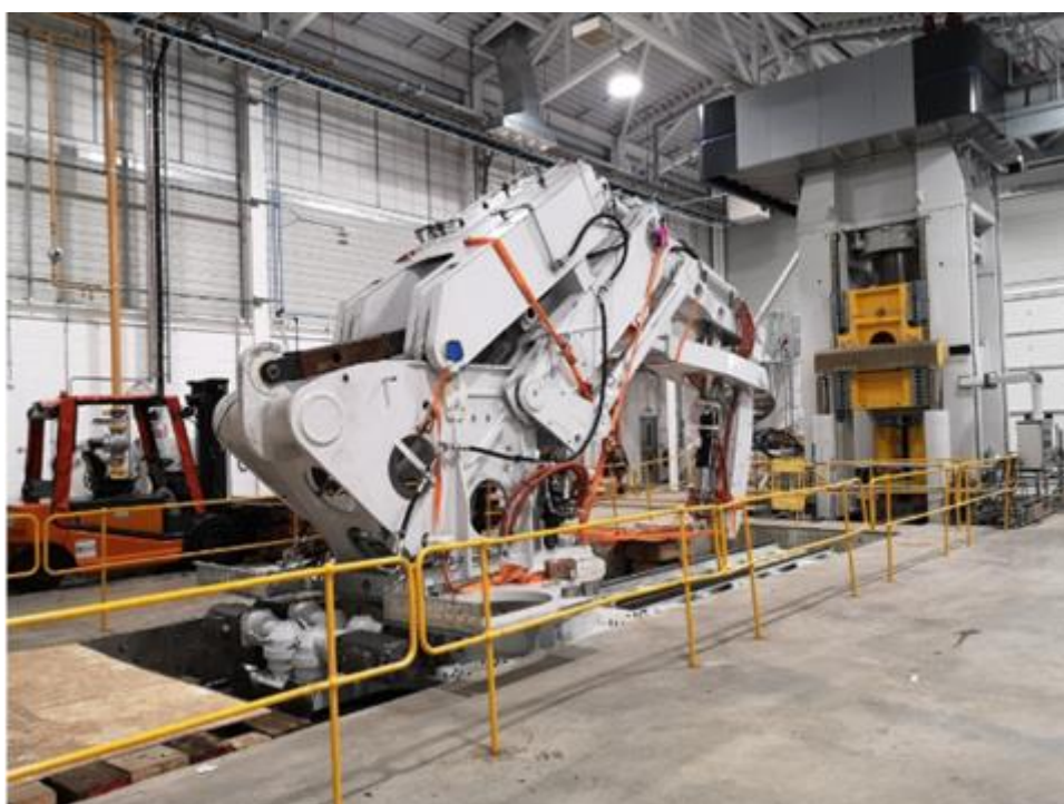
Figure 1: The FutureForge manipulator installed at the AFRC
