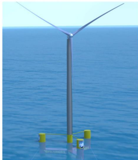
Figure 2. Image of the IEA 15MW reference turbine supported on the UMaine VoltturnUS-S reference platform [8].
