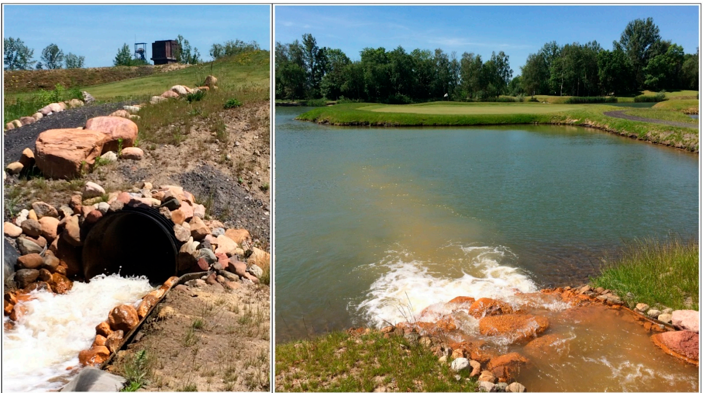
Figure 6. The pumped mine water discharge from Ewa shaft in Bytom, Poland ( left ), and its outfall into a lake within the ARMADA housing development complex ( right ). Reprinted with permission from ref. [70]. Copyright 2017 David Banks.
