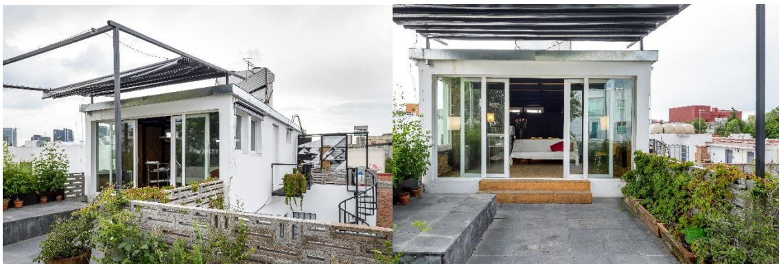
Figure 2: External views from the Passivhaus flat in Mexico City.
