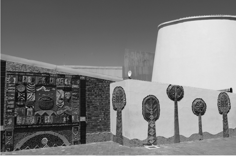
Figure 9.1 Street-front view of GugaS'thebe.
