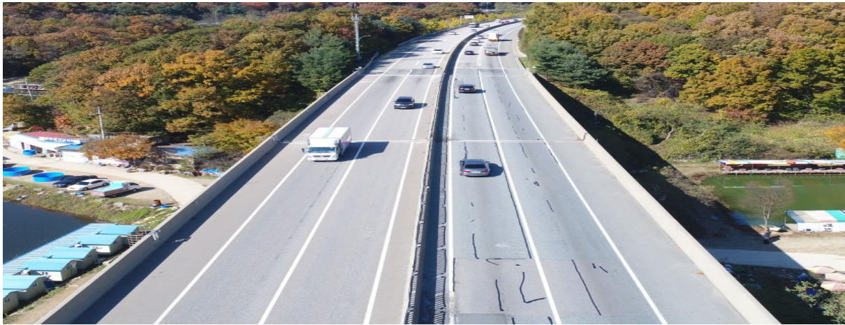
Fig. 2: Case study bridge
