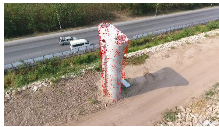
b) Features inside the pier from the proposed system
