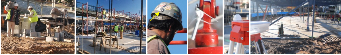
Fig. 2: Images of work environment (concrete masonry unit saw and columns), UWB tag on worker’s helmet and UWB tags on mobile crane hook, UWB reference tag on tripod and UWB receiver (from left to right image)
