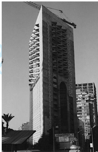
Fig 8. Faisal Bank Tower (source: by author).
