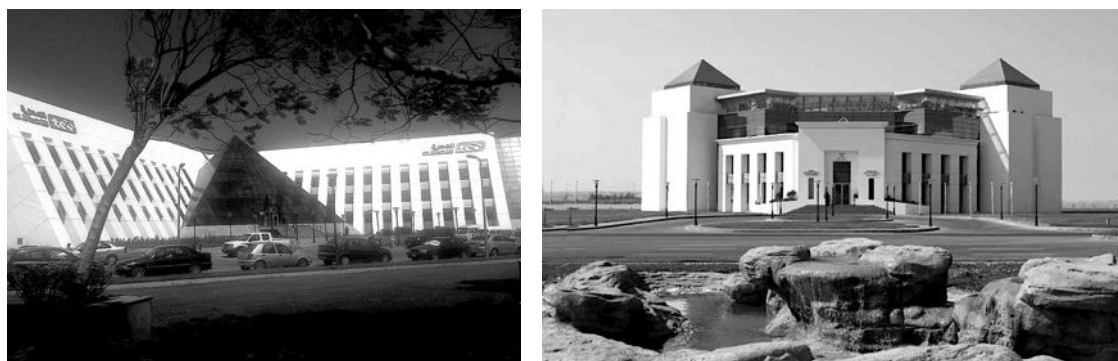
20 Fig 9. Left: Telecom Egypt (source: URL 5, 2014: by Mohamed Ouda); Right: CULTNAT 21 building (source: URL 6, 2010). 22
