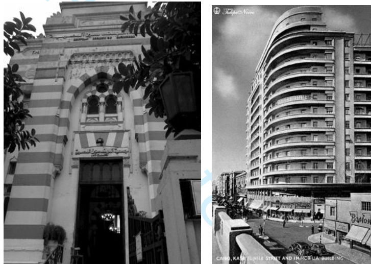
Fig 2. Left: The Society of Egyptian Engineers (source: by author); Right: The Immobilia Building (source: URL 1, 2012: by Tulipe Noire).
