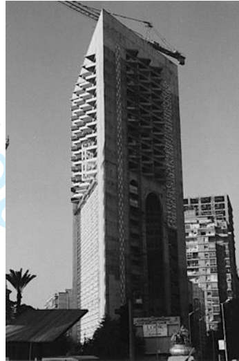
Fig 8. Faisal Bank Tower (source: by author).
