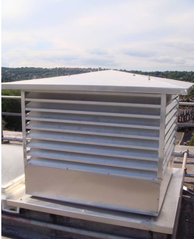
Figure 8 Experimental wind tower in situ
