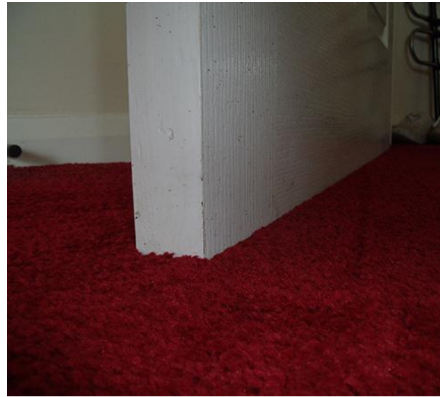
Door Undercut Blocked by Carpet
