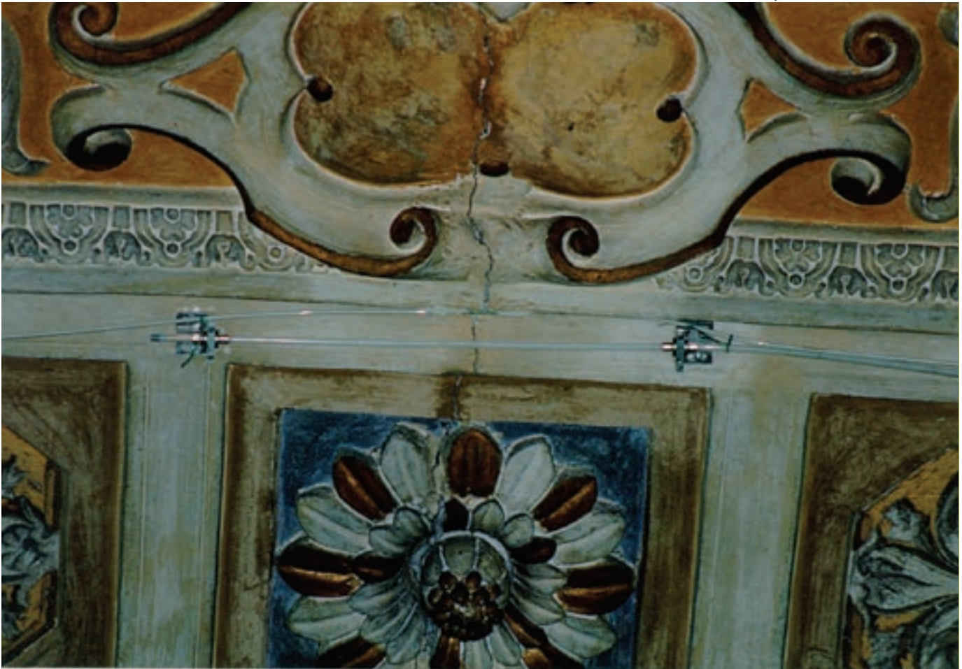
The SOFO displacement center shown here monitoring crack development in the 17 th century Gandria Church in Switzerland.
