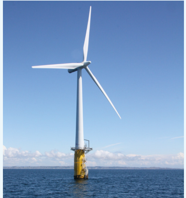
Figure 5: Equinor's 2.3 MW spar design; Karmøy, Norway (Source: DoE)
