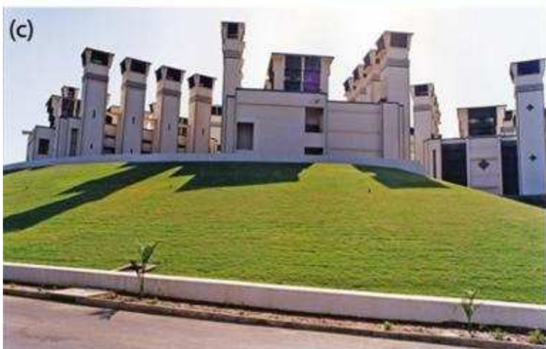
Fig. 9. Windcatchers in contemporary buildings: (a) Springs Preserve building in Las Vegas, USA; (b) Zion National Park Visitors Center in Utah, USA; (c) Torrent Research Center Building in Ahmedabad, India [65], [75] and [95].
