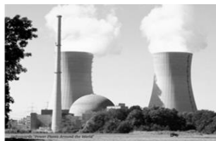
Nuclear Power Station
