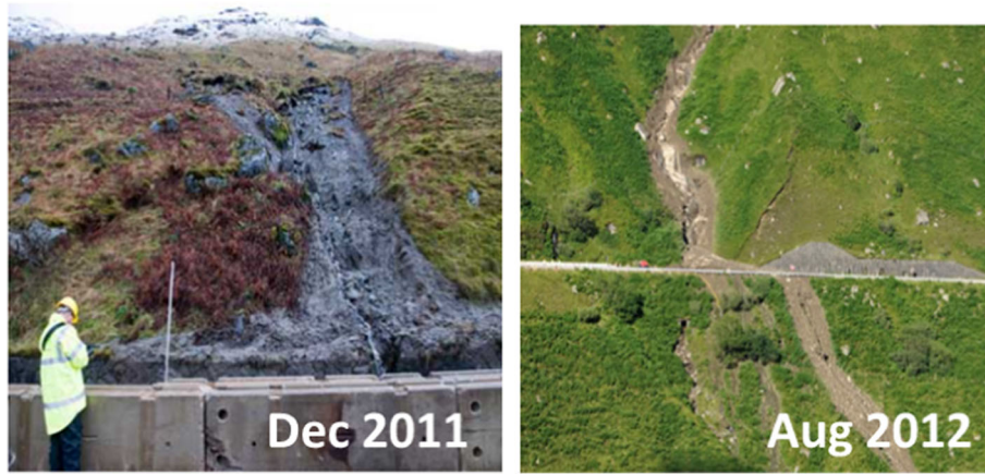
Fig. 4 December 2011 and August 2012 Landslide. BGS© NERC [2011]
