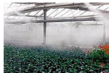
Figure 1b example of 'fog' production for greenhouse humidification using nozzles (Dutrie).
