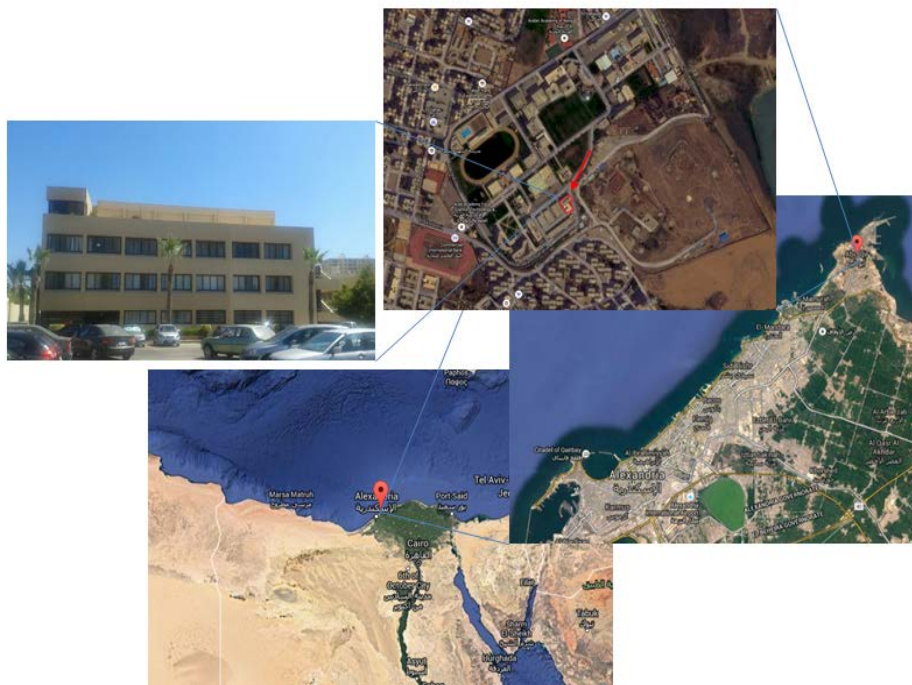
Figure 4. Location and external view of the office building.
