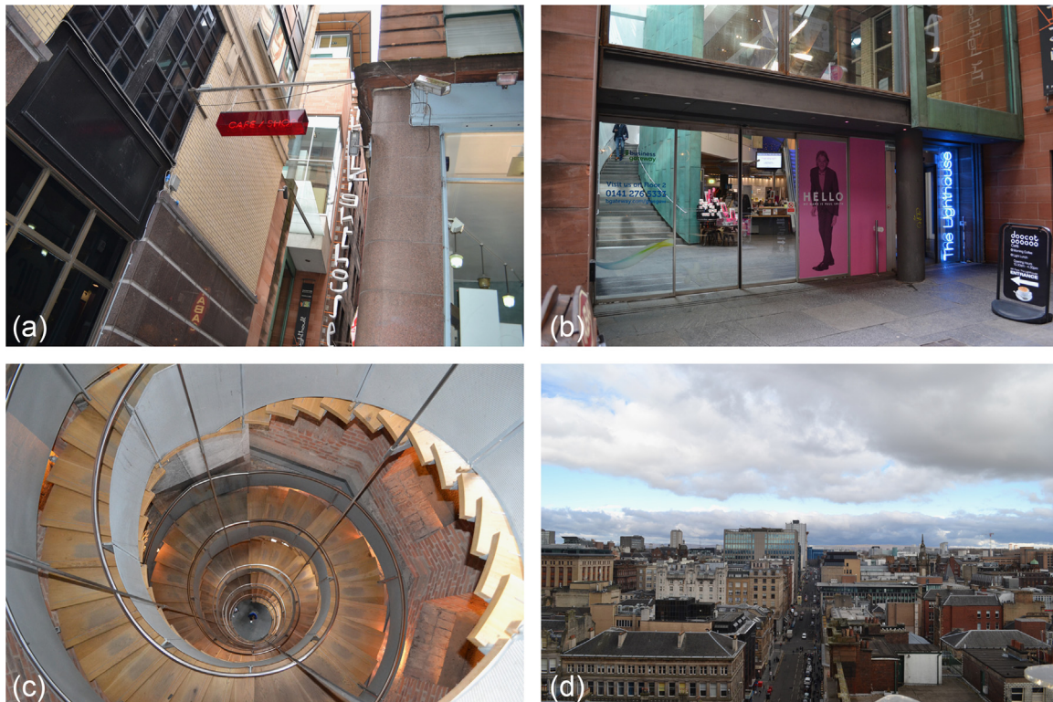
Fig. 4 The Lighthouse (Source: L. Maclean), (a) external, (b) entrance, (c) staircase, (d) first floor.
