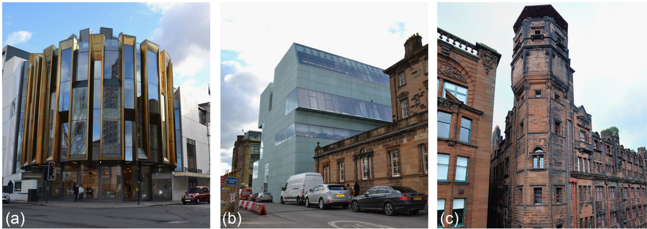
Fig. 1 Three buildings in Glasgow selected for assessment (Source: L. Maclean). (a) Theatre Royal , (b) Reid Building , (c) The Lighthouse .
