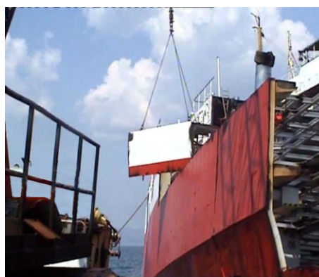
Figure 4: Mobile Crane in the Sea-Shore Interface
