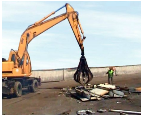
Figure 7: Poly-Grab Crane in the Secondary Zone
