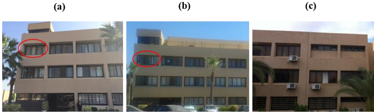
Figure 10. (a) Front side of the building on 07/10/14, (b) Front side of the building on 14/10/14, and (c) Back side of the building on 12/11/14.
