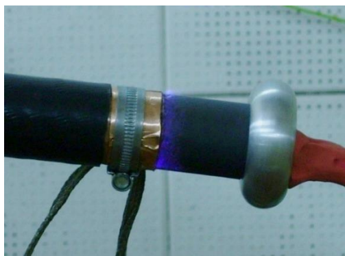
Figure 6. Defect type 5: Surface discharge around end termination.
