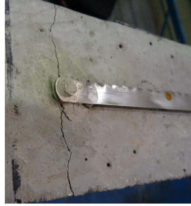
Figure 4. Photograph showing cracking of the beam at the grouted sensor anchorage.
