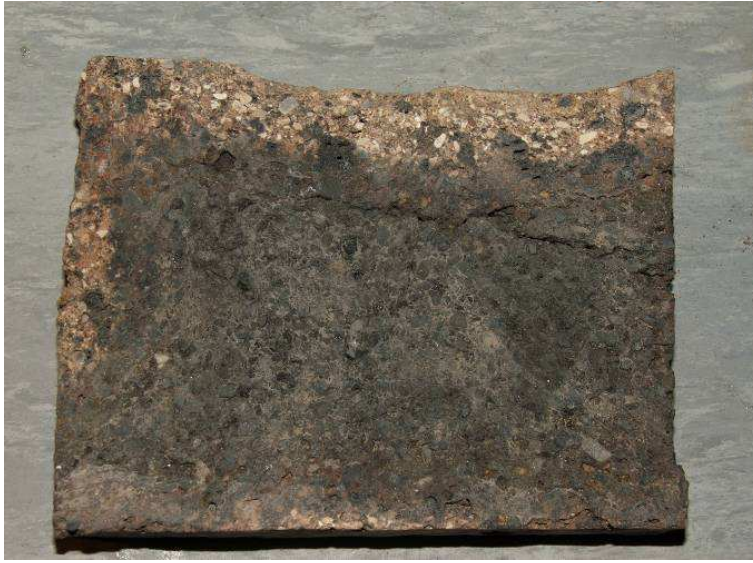
Fig. 4 Section through a Prestongrange brick (approximately 70 mm × 105 mm), viewed with the bed faces at the top and bottom, showing large horizontal cracks parallel to the bed face.
