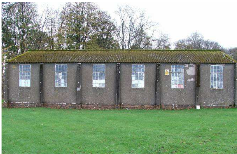
Fig. 2 A typical cement rendered brick masonry building at East Fortune airfield, East Lothian, Scotland. These buildings followed the standard designs produced during World War II by the Ministry of Defence, and were virtually identical to military buildings elsewhere in the UK [15,16]. The walls were built in stretcher bond, a half brick thick (about 120 mm), with brick piers at 3.3 m intervals, protruding both internally and externally.
