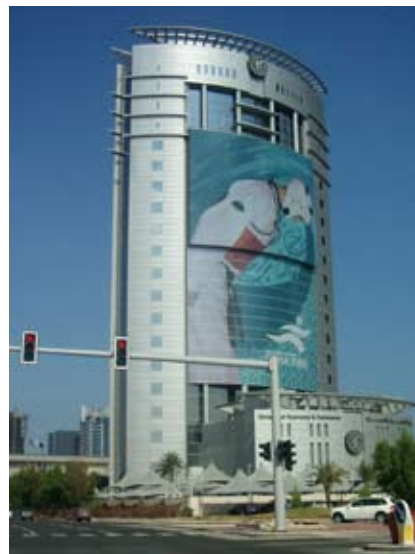
Figure 2: Headquarters of Ministry of Economy and Commerce, an example of Global Architecture.
