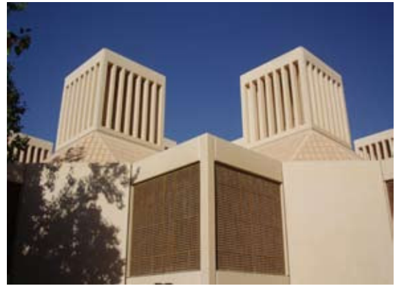
Figure 4: An attempt at establishing local identity, Qatar University campus.
