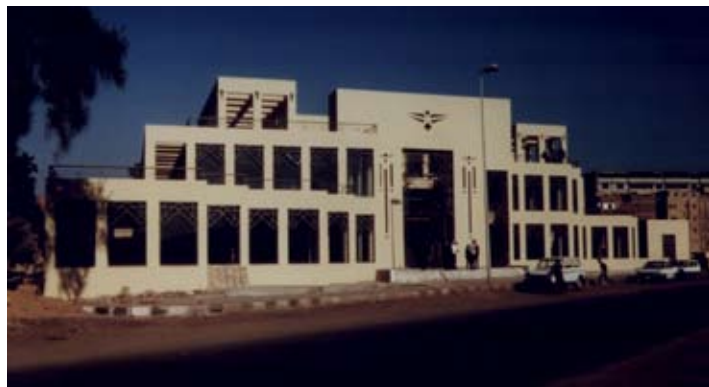
Figure 6: Commercial and Tourist Centre by Gamal Bakry. An example of Critical Regionalism — a conscious attempt at reinterpreting the heritage of Cairo.
