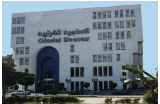
Figure 2: Original Weavers Company Headquarters by Farouk Al Gohary. An implicit example of historical revivalism.
