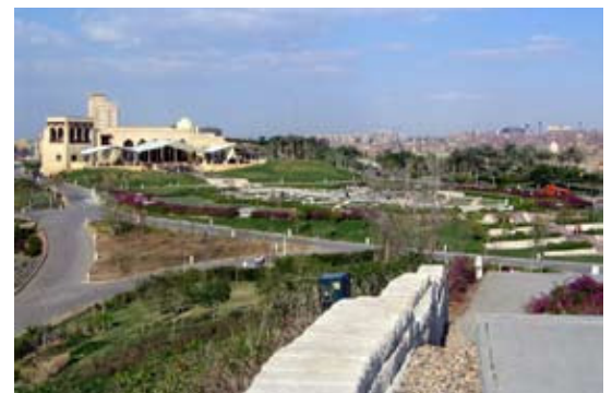
Figure 7: A view of Al Azhar Park: An example of culturally and environmentally responsive architecture.
