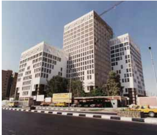
Figure 4: The Headquarters of the Ministry of Finance and Tax Department. Example of Surface Treatment Architecture "A Basic Design Exercise on Building Form and Facades," By Farouk Al Gohary. Photo: Arab Contractors
