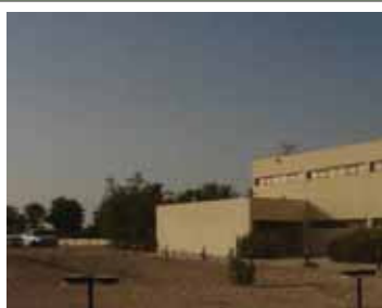
The space connecting the north uncovered parking lot with the back side of the library building
