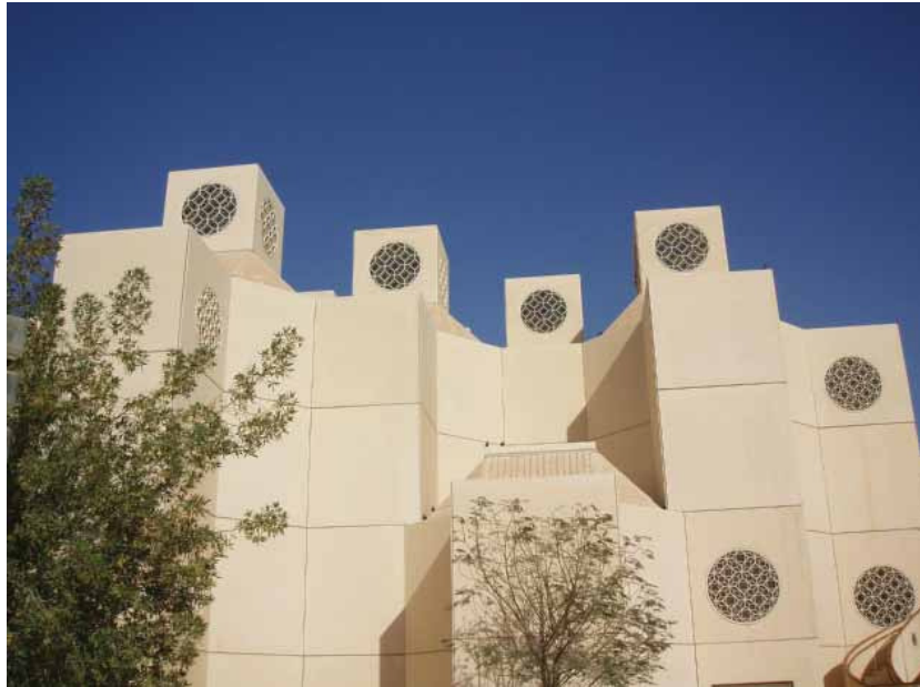
Figure 4.b: Emphasizing Natural Ventilation by Using Wind-Towers in the Education Technology Center. (Source: Author).
