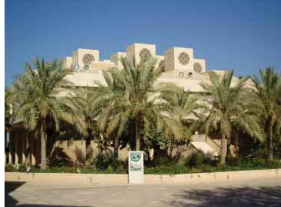
Figure 4.a: Utilization of Wind Towers in Main Administration Building of Qatar University. (Source: Author).
