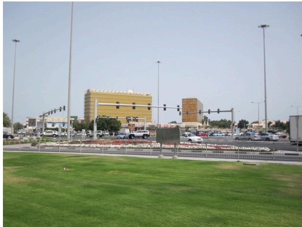
Figure 8: Ramada Junction. (Source: Authors).
