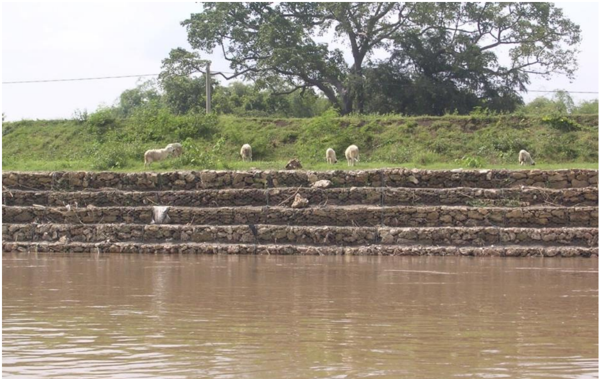
Figure 2. Two-step man-made embankment with surface protection in the form of rock filled gabions.
