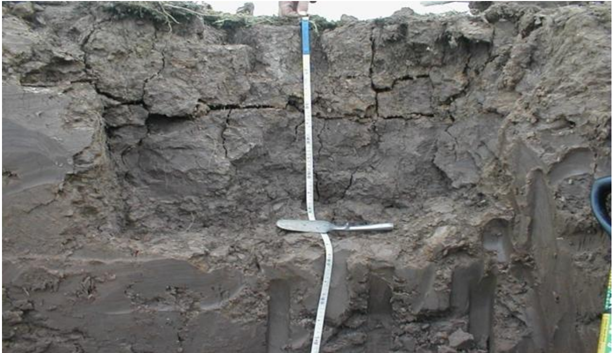
Figure 1. Exposed fissures through trenching on the disused Thorngumbald embankment (after Dyer et al. 2009).
