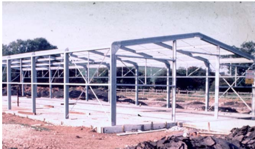
Figure 1: Cold-formed steel portal framing system
